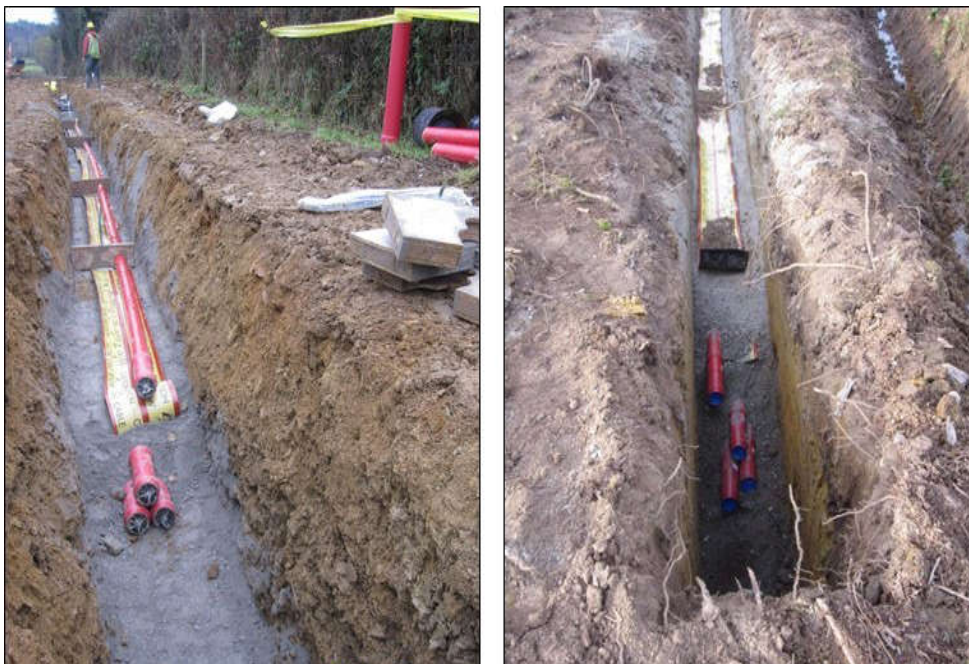
Plate 2-1 Typical Cable Trench View
